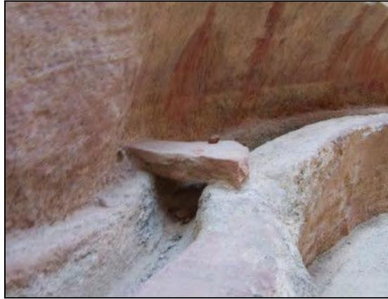
The longest canalisation goes up to 3 km, the biggest cisterns were up to 7 meters deep with a diameter of 6 meters. The cisterns collecting rainwater were provided with spillways, allowing the excess of water in the upper cistern to flow into the lower one. Water was also filtered with the help of sedimentation basins. All the hydraulic apparatus was characterized by the simplicity of the techniques adopted and by flexibility in management.
